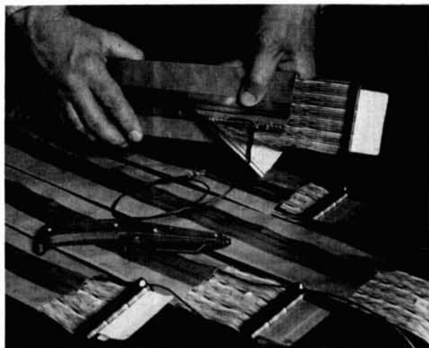
fig. 13. Zippertubing conductive cable covers for suppression of conducted interference.
